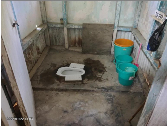
Toilet in doctor room
