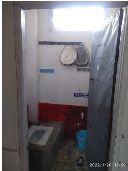
Repair of toilets
